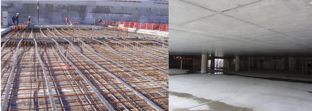
Figure 1.10. Prestressed concrete parking lot floor
