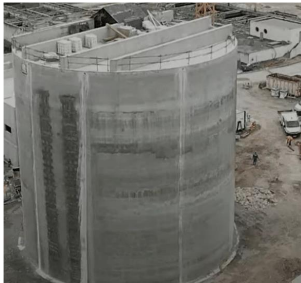
Figure 1.11. Prestressed concrete reservoir
