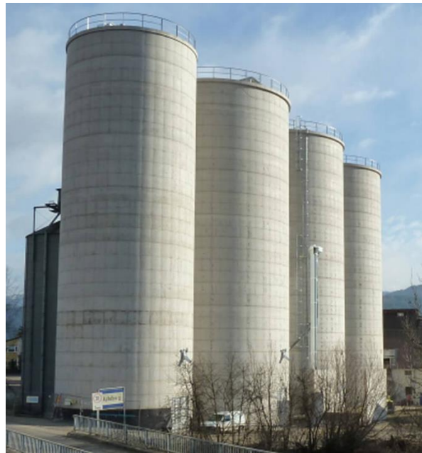
Figure 1.14. Prestressed concrete silos
