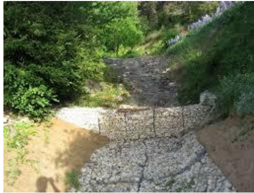
Figure 2.2. Seuil en gabions.
